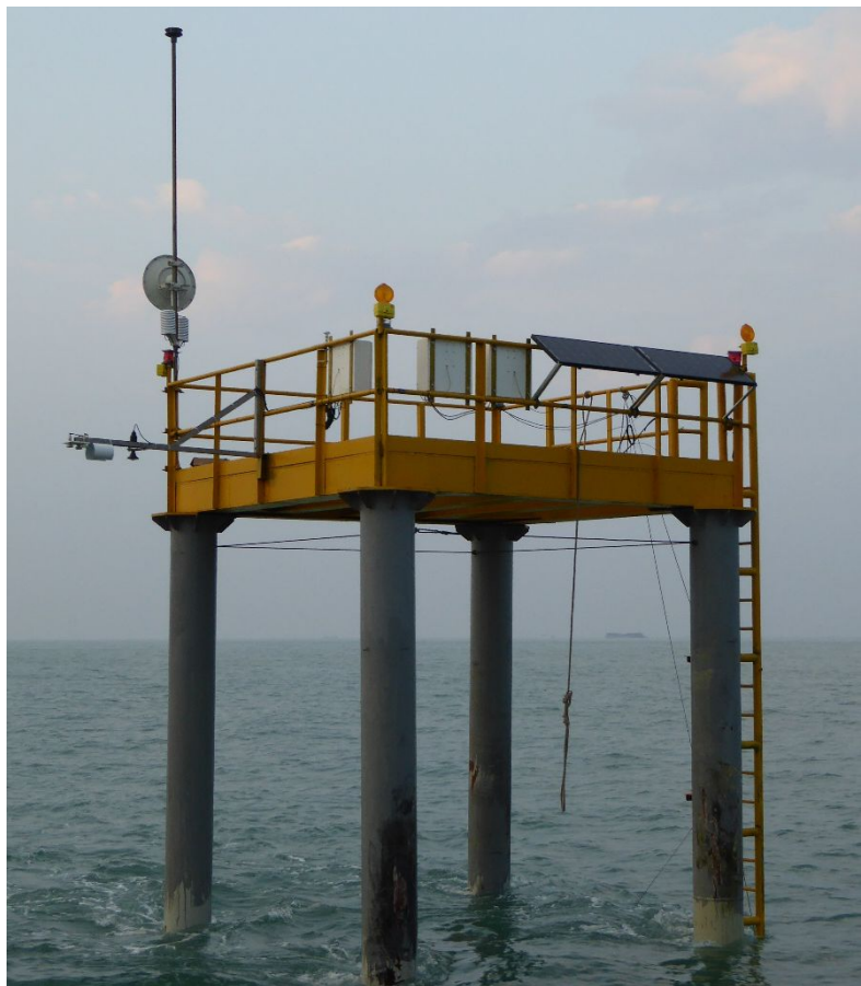
The platform after installation
